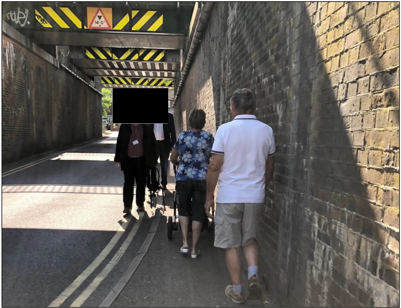
Figure 62 Pedestrian congestion under railway bridge
